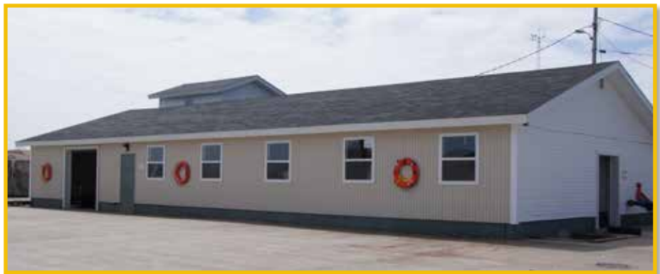
The renovated former fish plant in Lord's Cove.
